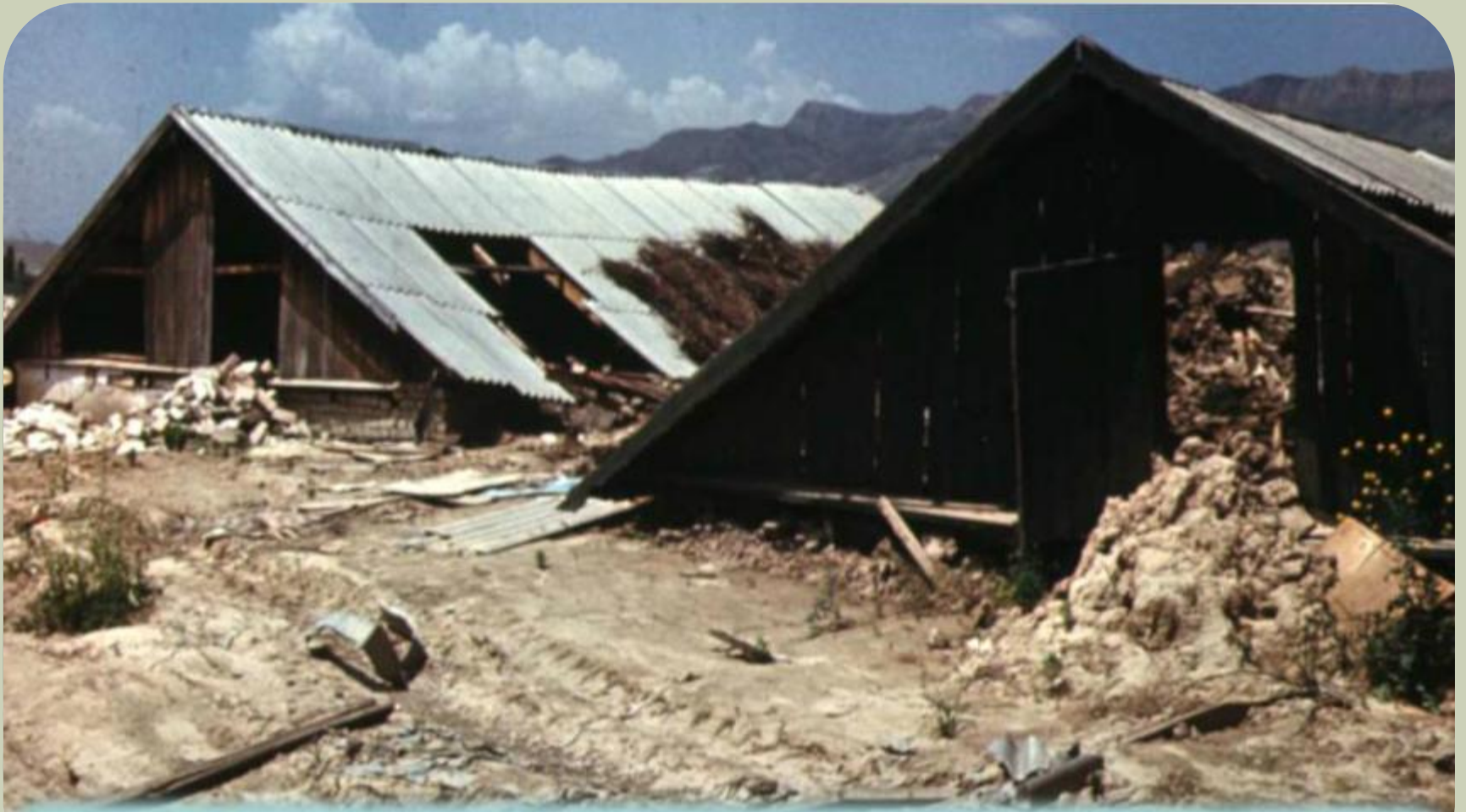
Houses, flooded by a landslide after Hissar earthquake 23/01/1989
